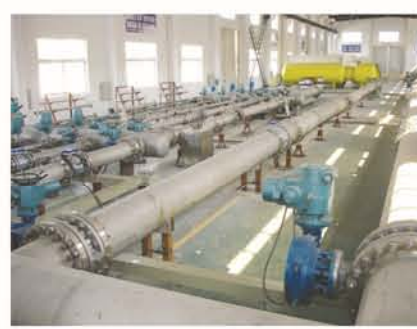
Flow Resistance Testing
